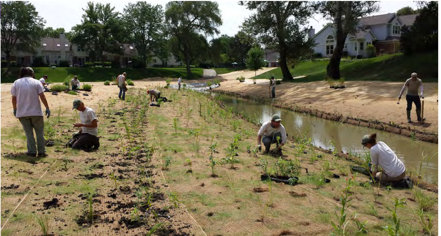
Proposed plug planting through erosion control fabric after seeding.
