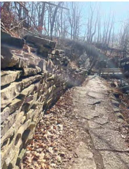
Existing leaning stone wall to be rebuilt.
