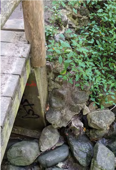
Existing exposed bridge foundation.
