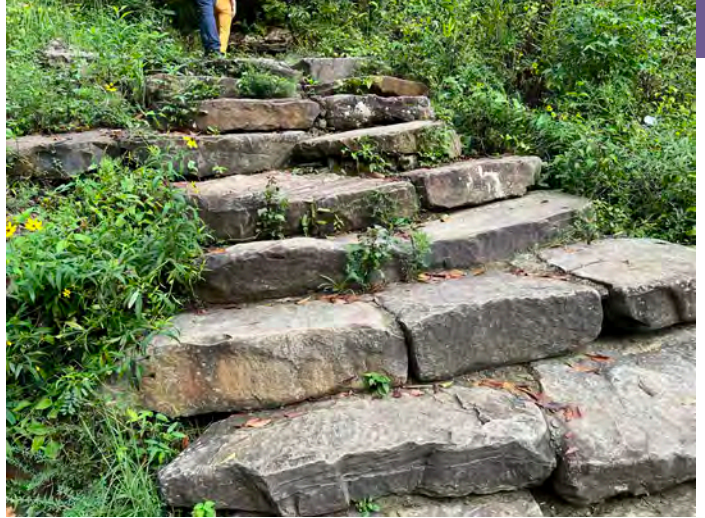
Example water access: Stacked outcropping stone at key points along stream.
