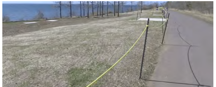
Example temporary stake and rope fence to protect restoration areas.
