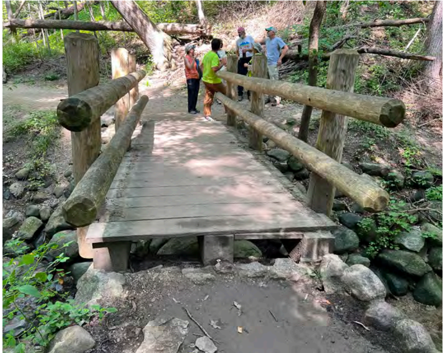
Uneven trail and bridge surface with muddy landing area where a boardwalk connection is proposed.
