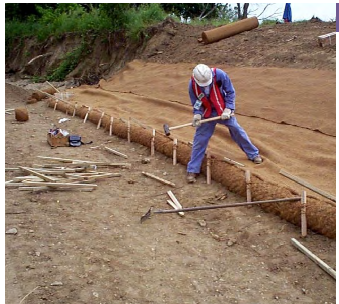
Proposed erosion control approach with erosion control fabric and coir logs.
