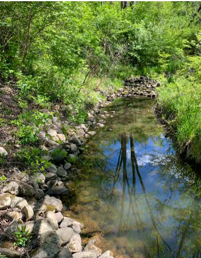
Example stream condition: Natural stone toe protection and riffle in-stream structure.
