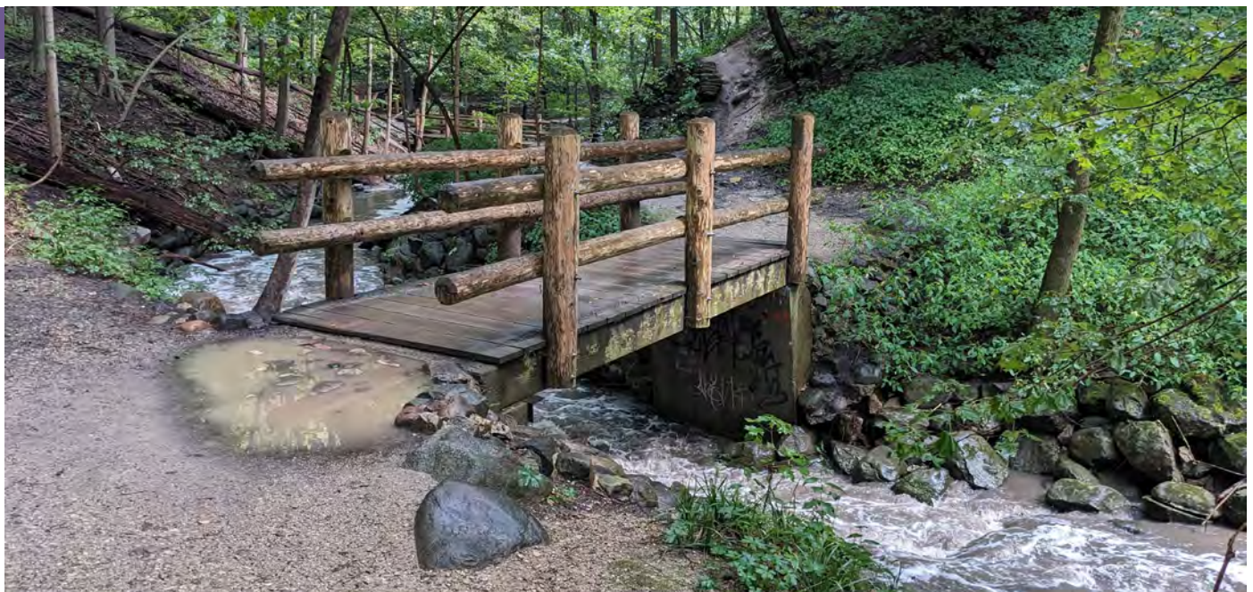
Erosion around bridge foundations and turbid water after a storm.
