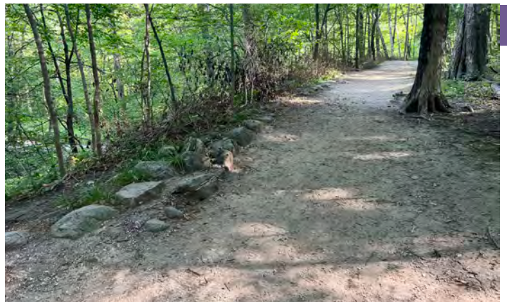
Existing trail with boulder edge protecting slope vegetation and opposite side without edging expanding.
