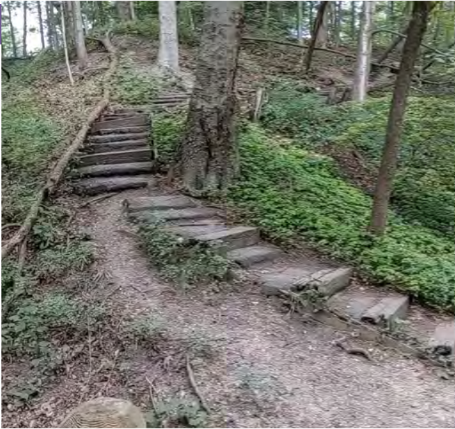
Existing timber stair in disrepair to be removed.
