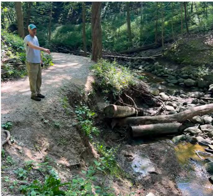
Bank erosion threatening an adjacent trail that serves as the main access path to the beach shown at low water level and immediately after a short storm.
