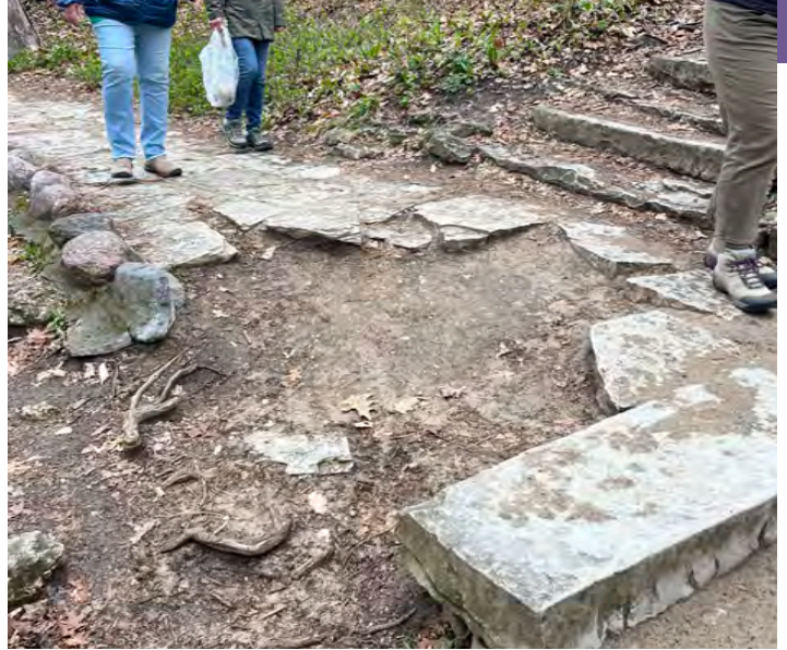
Existing stair landing with missing lannon stone paving and adjacent wash-out.
